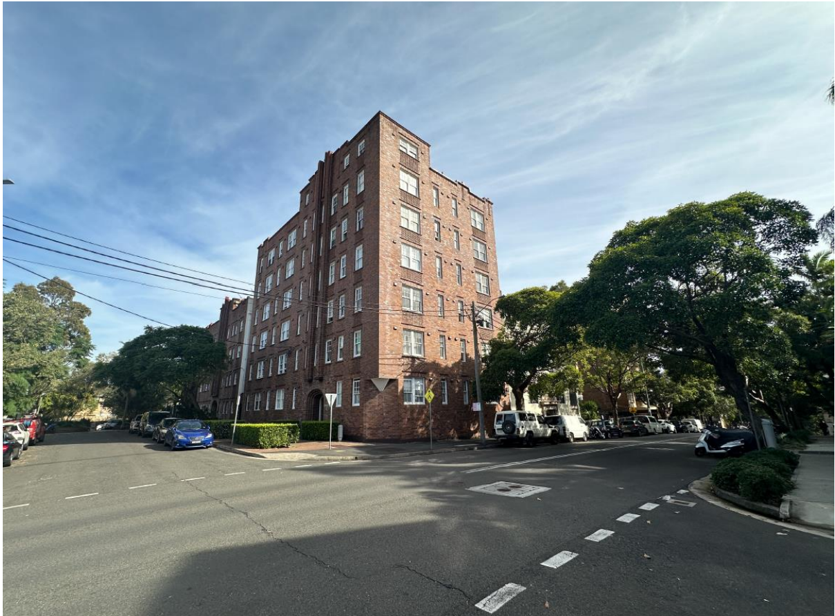
Figure 4: Looking south-west from the Liverpool Street and Darley Street intersection towards the neighbouring residential flat building of 3-5 Darley Street, situated to the east of the site (subject site is situated on the right hand side of 3-5 Darley Street and hidden behind street trees)
