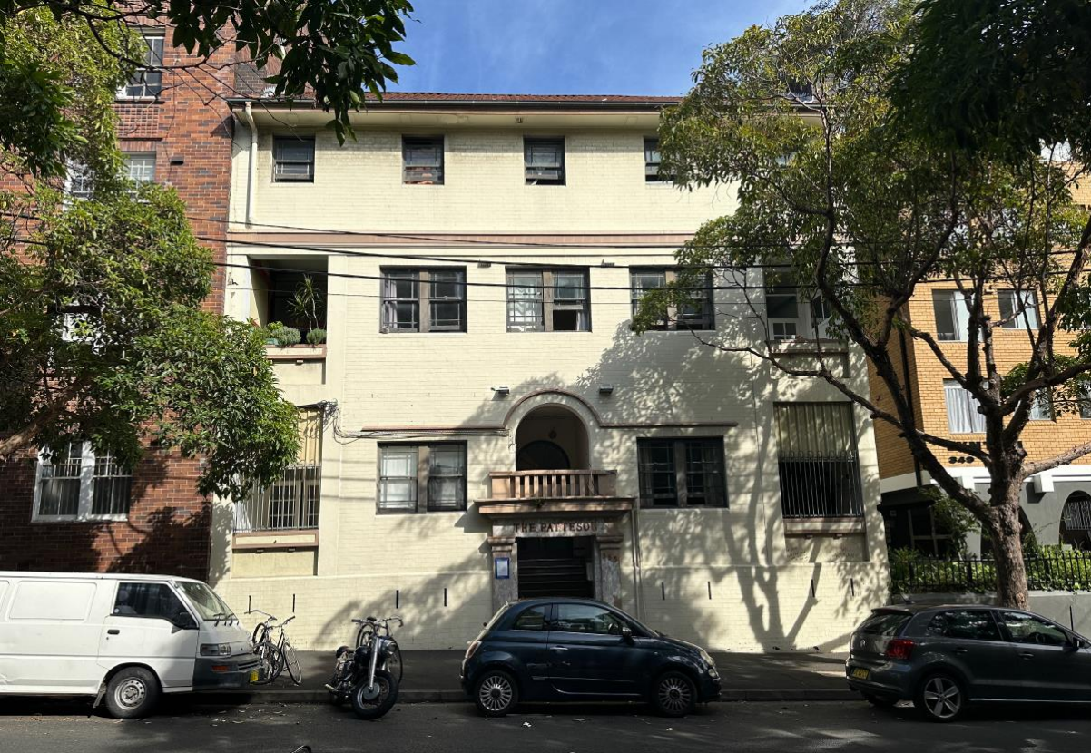
Figure 2: Front of the site viewed from Liverpool Street
