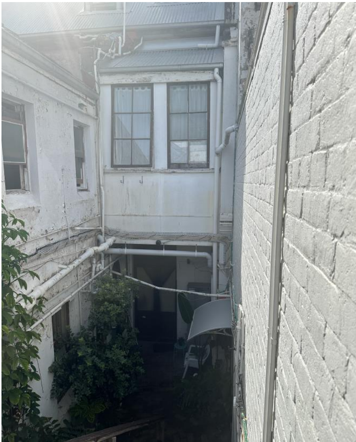
Figure 12: Existing internal courtyard of subject site
