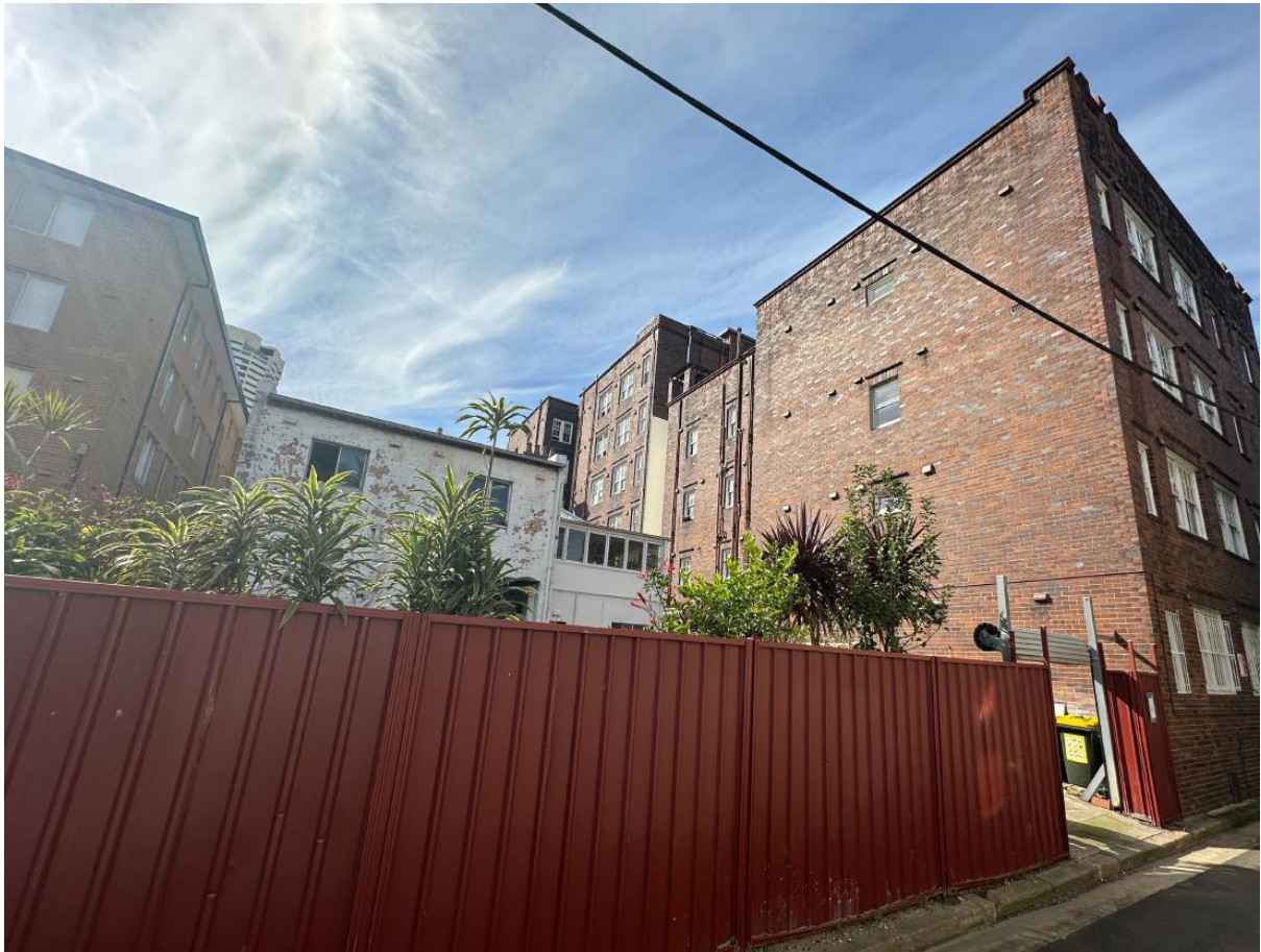
Figure 5: Rear of the site viewed from Darley Street
